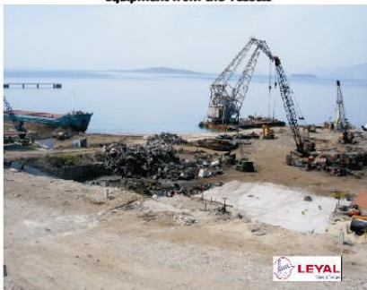
Floating crane facilitates the removal of heavy equipment from the vessels
