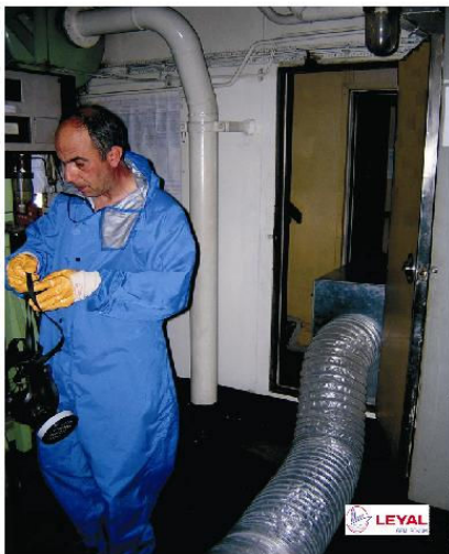
Negative pressure chamber is setup prior to asbestos removal operation
