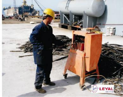
Cable sheathing is removed and disposed of appropriately
