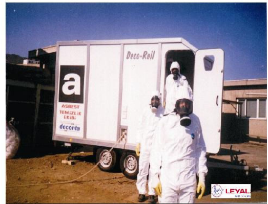
Waste removal team proceeding to work area
