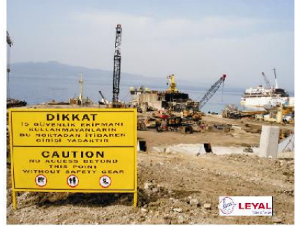
Ship dismantling work area
