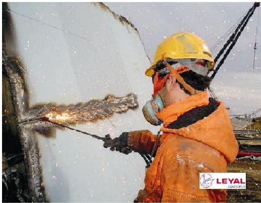
Torch cutting of steel plate
