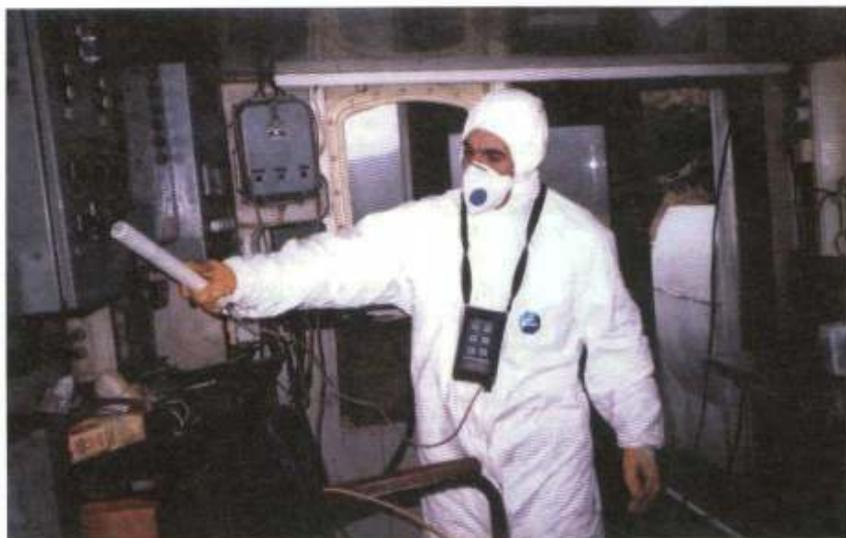
Gas free and radiation checks are integral parts of the pre-demolition assessment of the vessel
